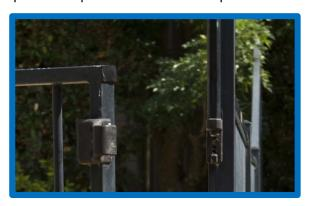
2. Gates and doors that are no longer self-latching General wear and tear of the locking mechanism means that many gates and doors will no longer self-latch when they close. If the gate or door is not properly locked, children may be able to gain unsupervised access into the water area.
