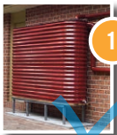
1 A water tank for topping up the pool
